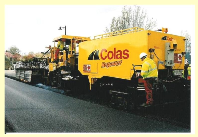
Surface heated, scarified, re-profiled, new thin overlay superimposed in one pass
