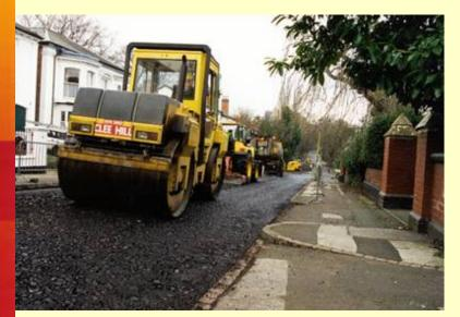
New emulsion binder added & compacted 14mm dry stone rolled in
