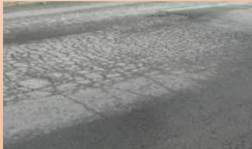
Alligator cracking due to
