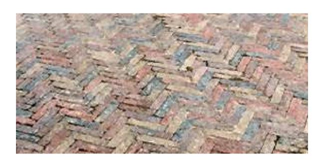
In the Netherlands the lack of natural stone led to the use of clay pavers to create their roads. Standard pavers (225x50x90) were used, laid on edge in a thin 4x4 herringbone format.
