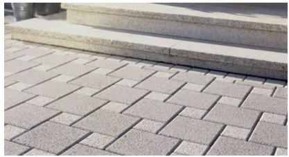
Bush Hammering both exposes the aggregate and fractures its top surfaces
