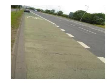
HFS – Short laying period, low durability, tendency to delaminate
