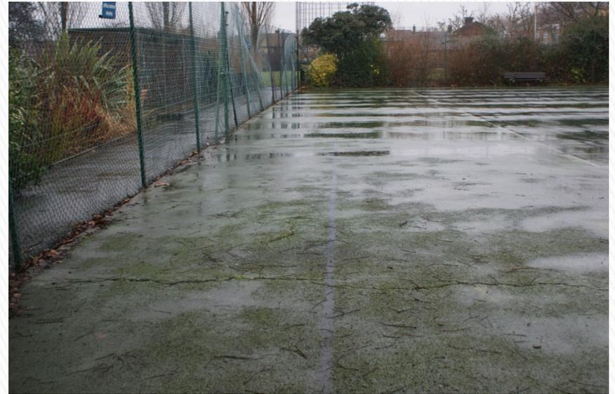
Undulations, loss of porosity and cracking– not usual macadam's fault
