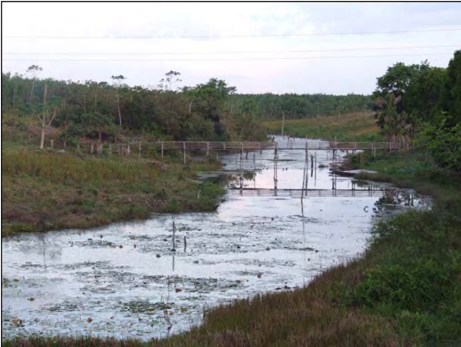
Spot # 23. APP along the State Road PA 150, showing the degradation of the riparian forest.
