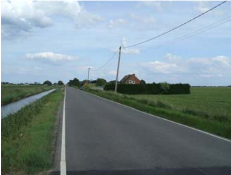
Condition after 4 years (June 2008)
