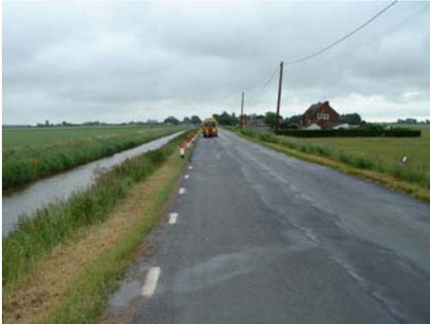
Prior to Works (August 2004)
