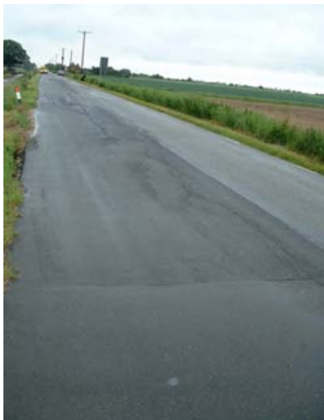
Prior to Works (August 2004)
