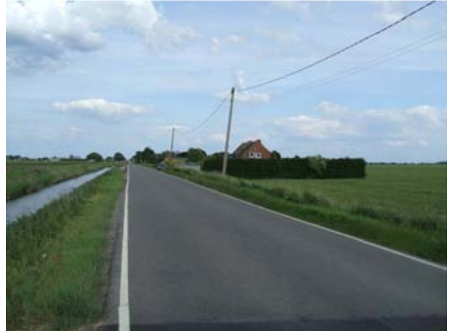
Condition after 4 years (June 2008)
