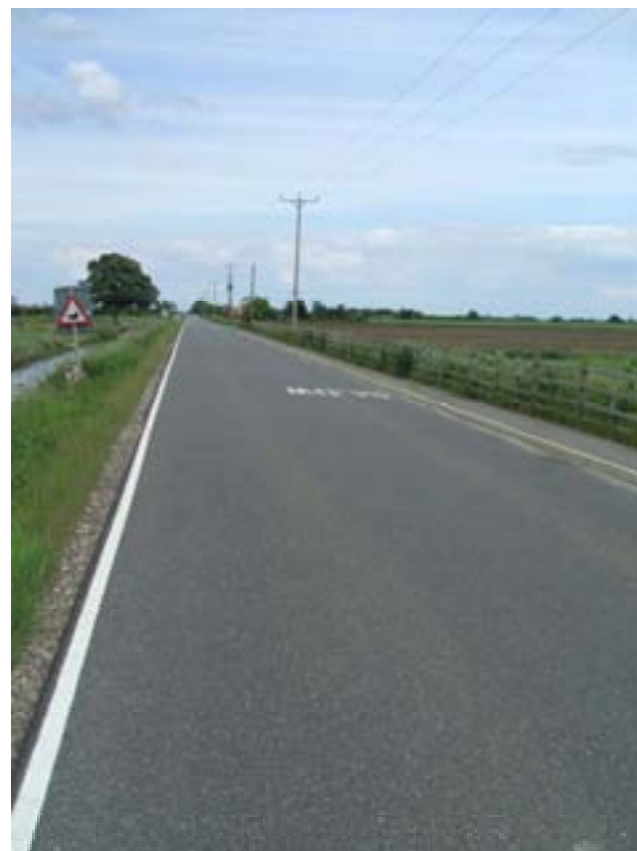
Condition after 4 years (June 2008)
