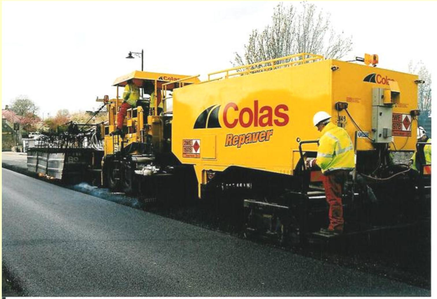
Surface heated, scarified, re-profiled, new thin overlay superimposed in one pass
