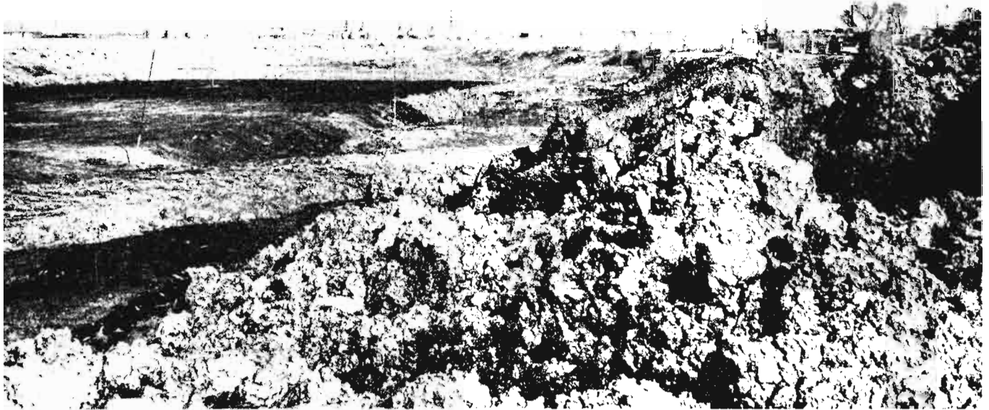
Above: The licenced tip between the old and new river walls will take 350 000 m 3 of fill. The inner slope on the river side is stabilized with interlocking concrete blocks (below, left) which will be removed as the tip is filled to avoid interference with future piling
