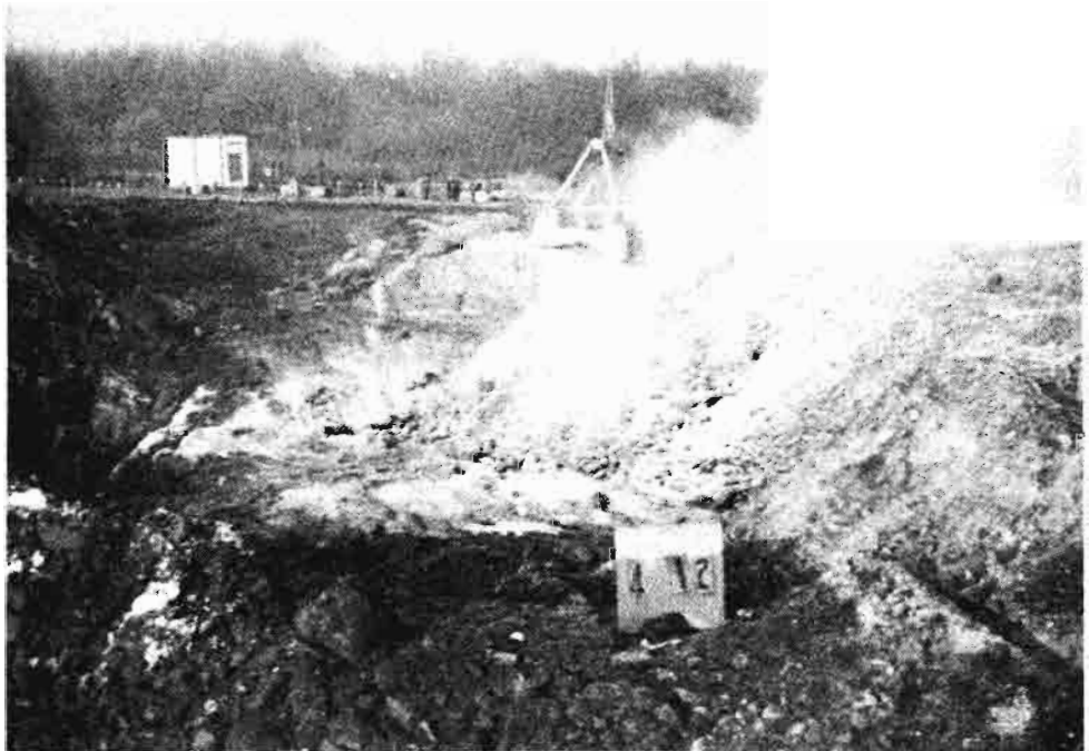
Ravenfield Tip - Treated materials being deposited in the quarry. The steam and lime dust can be seen rising from the heap.
