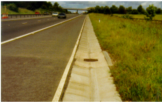
Figure 2: A typical scene of surface water channel drain and a layout of its construction.
